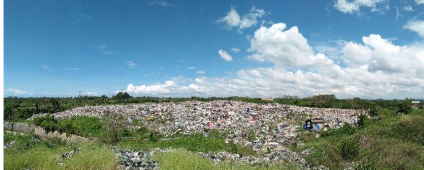
Gambar 1. Sistem Open Dumping TPA Temesi Sumber : Survey (2021)
